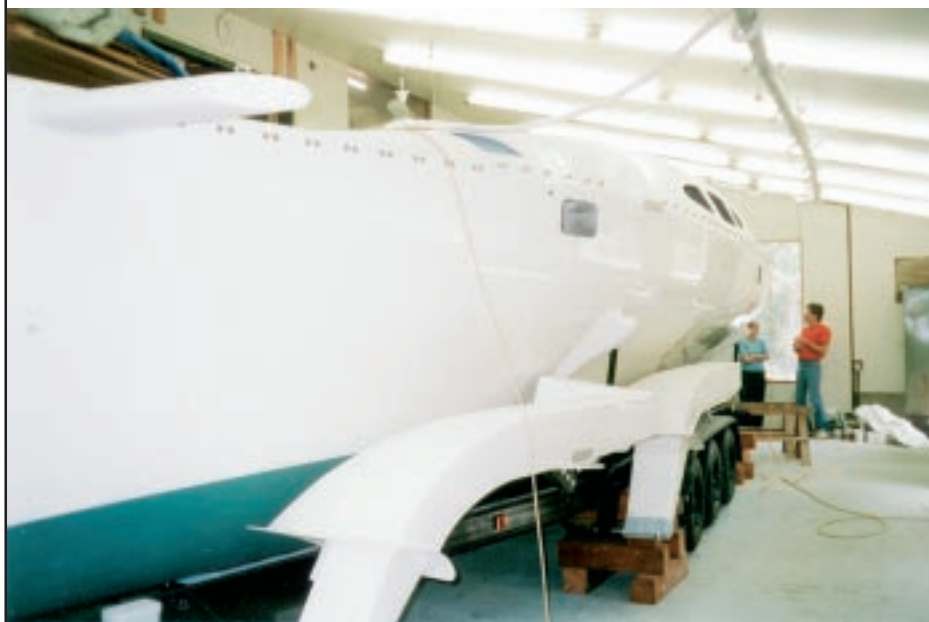
Scott Webster's F-36 having just been fitted to its trailer, and in the process of final fitout. Beams are mounted on the side of the trailer while floats will go on top. Being built by Andy and Mark Webster, the workmanship is superb. Note the bow wing which allows wider bow nets. Over 30 F-36's are now building.
